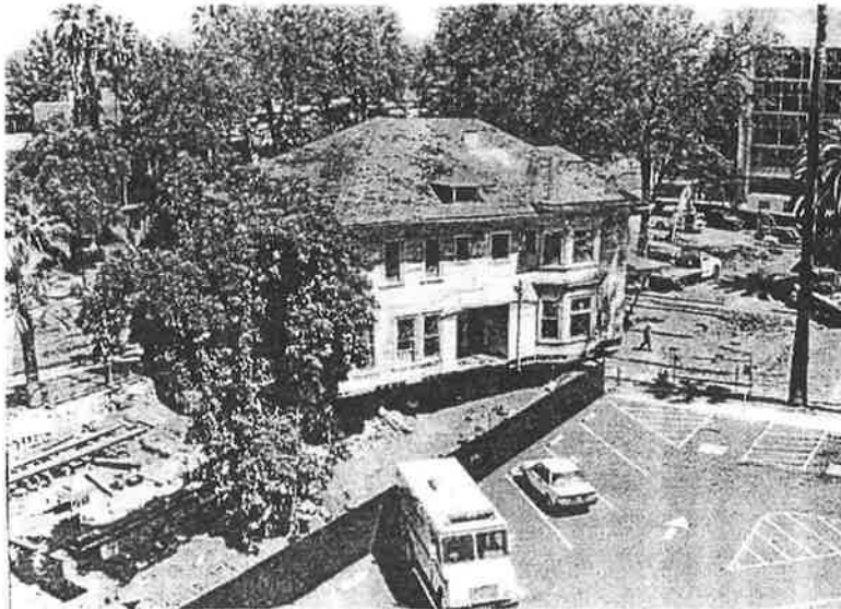
View from the top of Fourth Street Garage as the Scheller House is rotated and moved.
