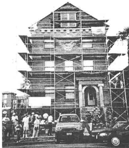
Scaffolding surrounds 311 N. Second Street
