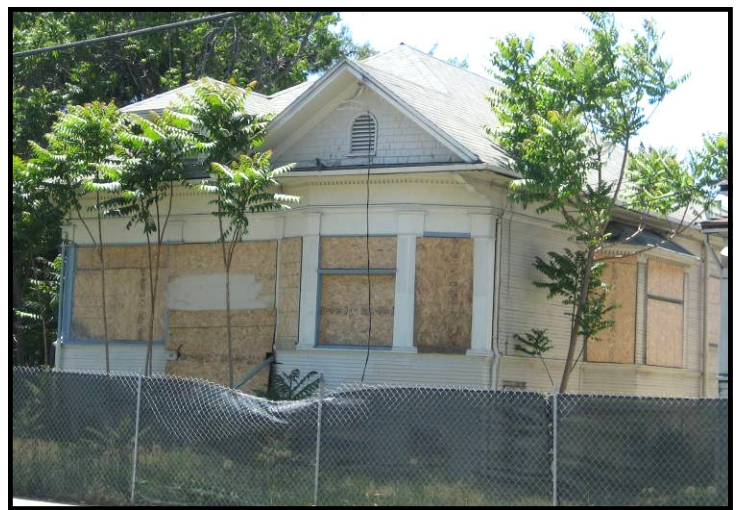
The Peschal House at 255 Delmas Avenue
