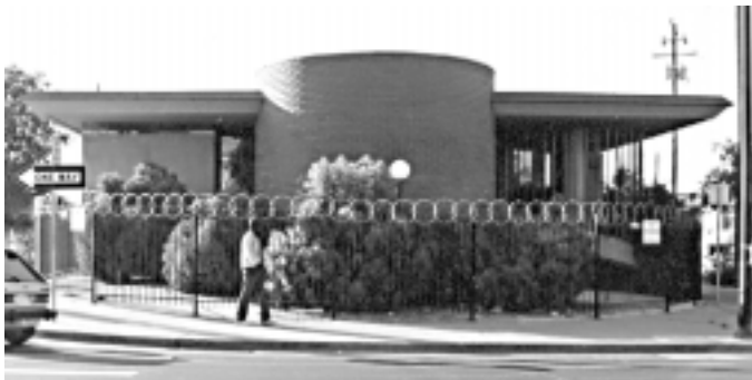
Weir Building, demolished in early 1990s
