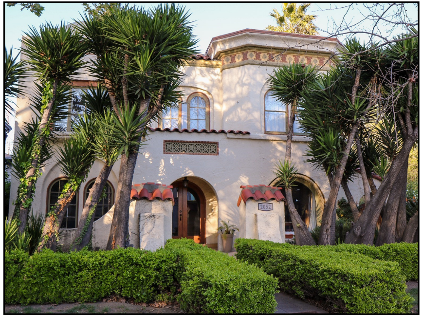
This distinctive Alameda Manor house was the home of O. Edwin and Ida Linquist of the Linquist Grain Company.
