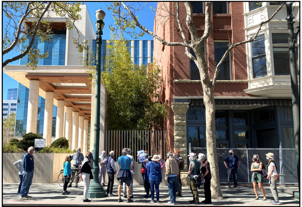
Walking Tour guests view the Moir Building next to the newer Federal Courthouse; its design respects the historic buildings in St. James Historic District. (Photo Ben Leech)
