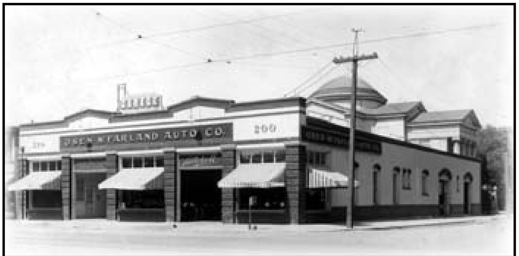
Letcher's second garage on the corner of North First and St. James Street. In 1907 Letcher sold the garage to Osen & Hunter (later becoming Osen & McFarland).
