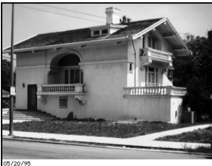
Gates/Maybeck house in 1995
