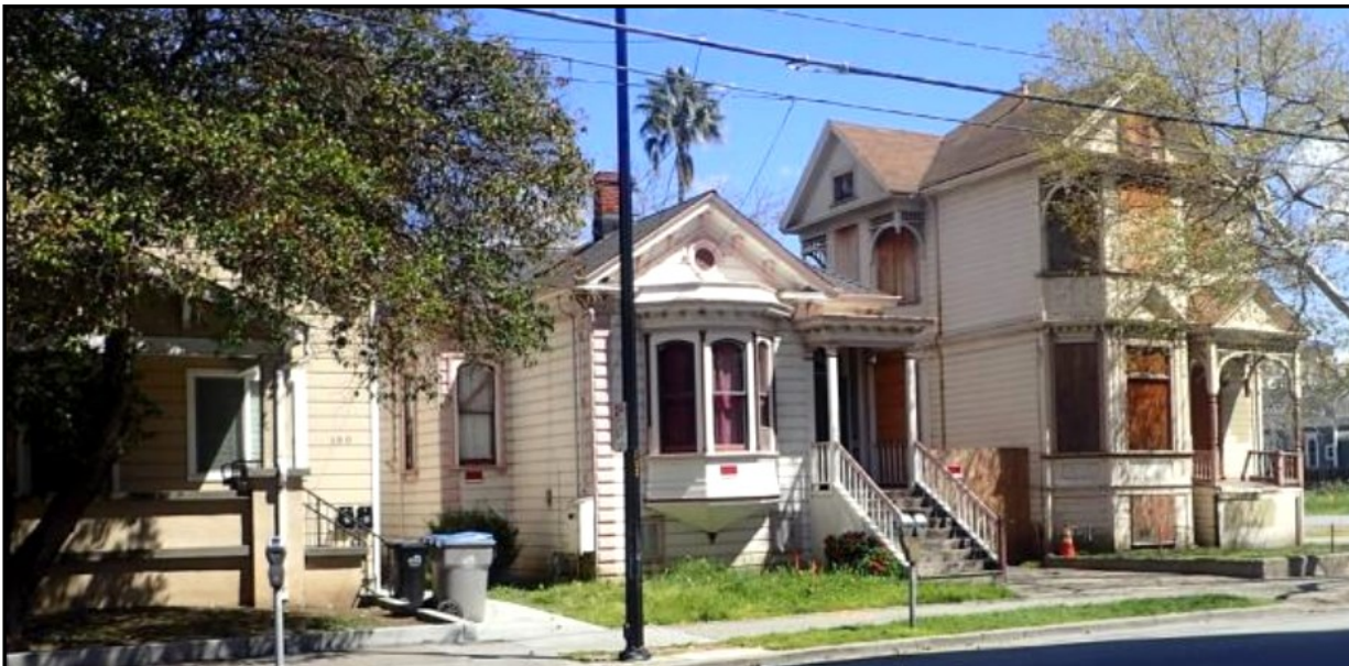
Houses from left, occupied house saved, middle house at 152 N. 4 th , and house on right at 146 N. 4 th Street, both destroyed by fire.
