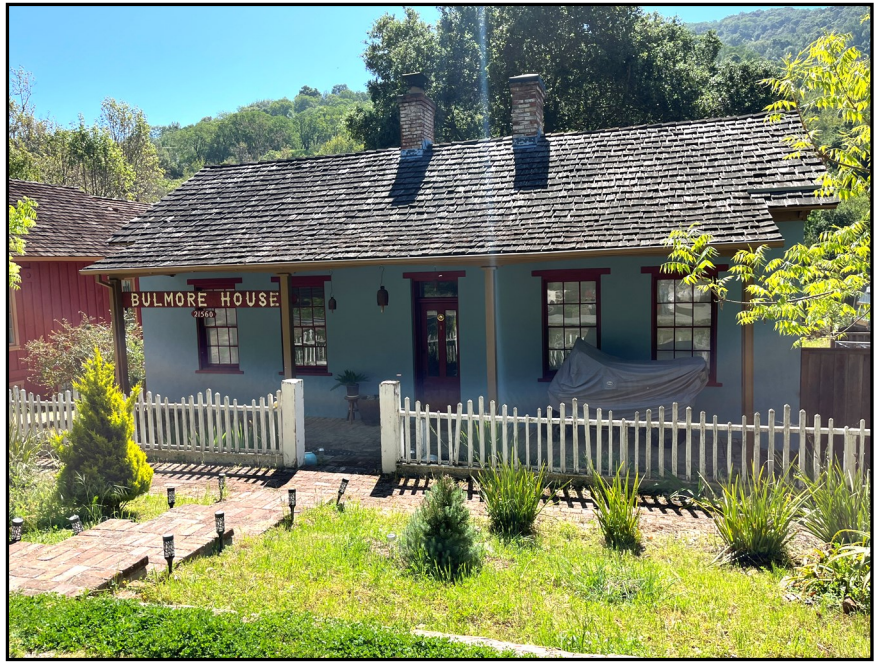
The Bulmore House was the first cottage built with locally produced bricks in 1854. Robert Bulmore and family lived here. He was last mining manager and last official resident of Casa Grande. His son, Laurence Bulmore, authored the book, Cinnebar Hills.
