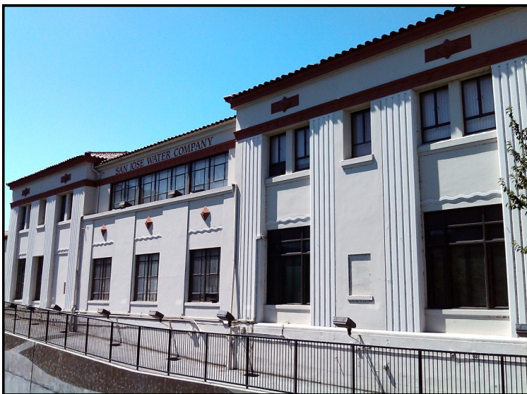
East view of SJWC building, facing Guadalupe River, taken in 2013 (Gayle Frank).
