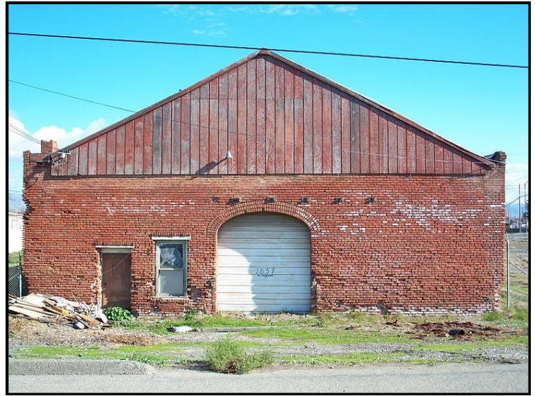
Front of Wade Warehouse.
