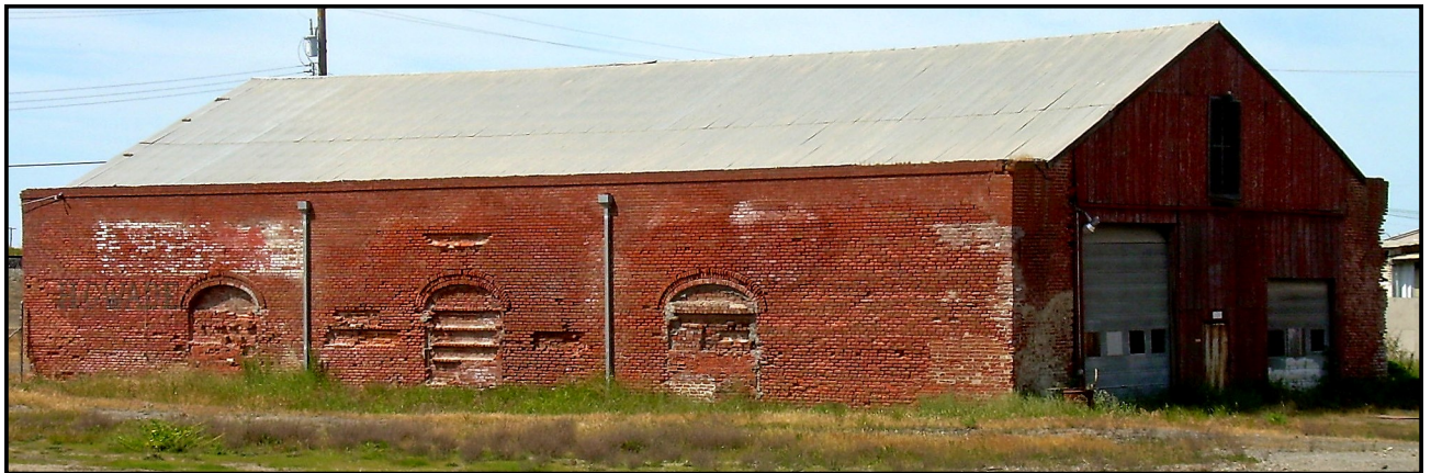
Above: rear/side view of the Wade Warehouse.
